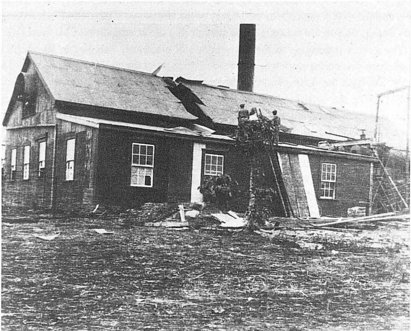
The original Bulawayo power station, 1897-1923. The damage seen in the picture was caused by a bursting flywheel following an engine overspeed.
