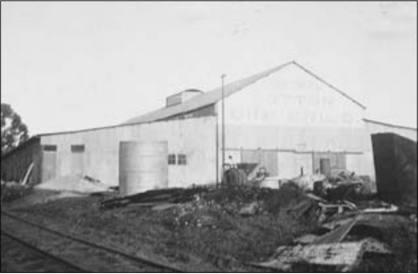
Meikles old store house – first Bata factory premises in Gwelo (1939)
