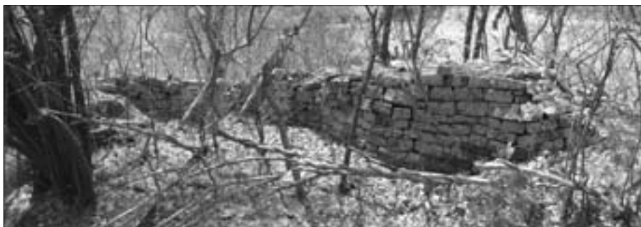
Fig. 1. “Q-type” walling. Northeast inner wall
