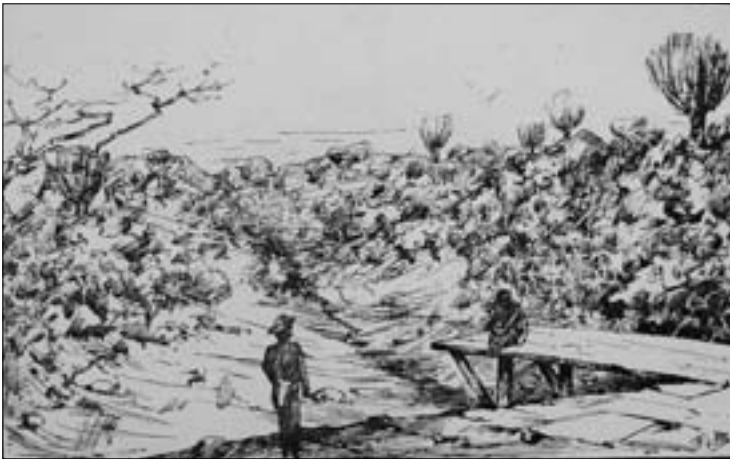
Fig. 2: Dam Number 2. Bulawayo Sketch 28/3/1896. Now lost after failing in January 1898.
