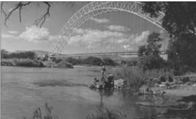
The beautiful Birchenough Bridge – southern gateway to the Eastern Highlands
