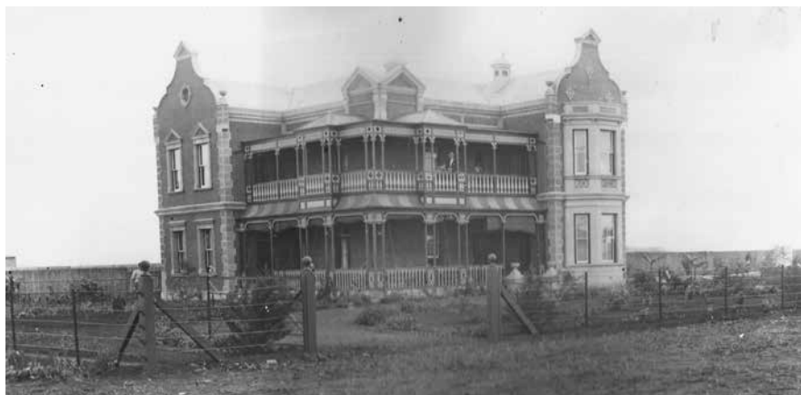
Johnson's first house in Salisbury in the Avenues
