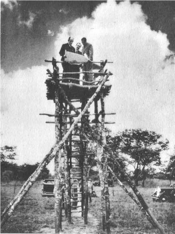
Prince George, Governor Young and architect John Hoogsterp surveying progress in 1934
