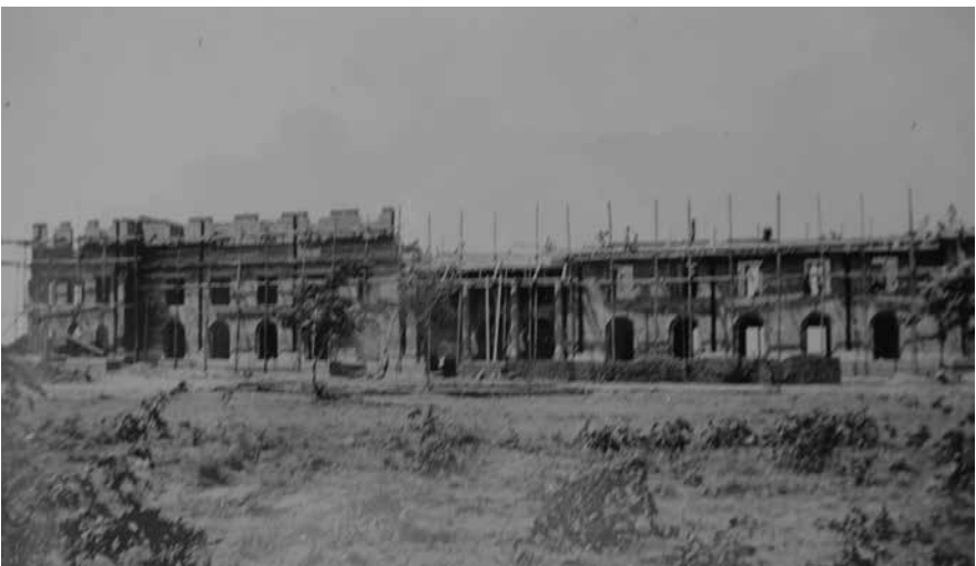
The Secretariat under Construction
