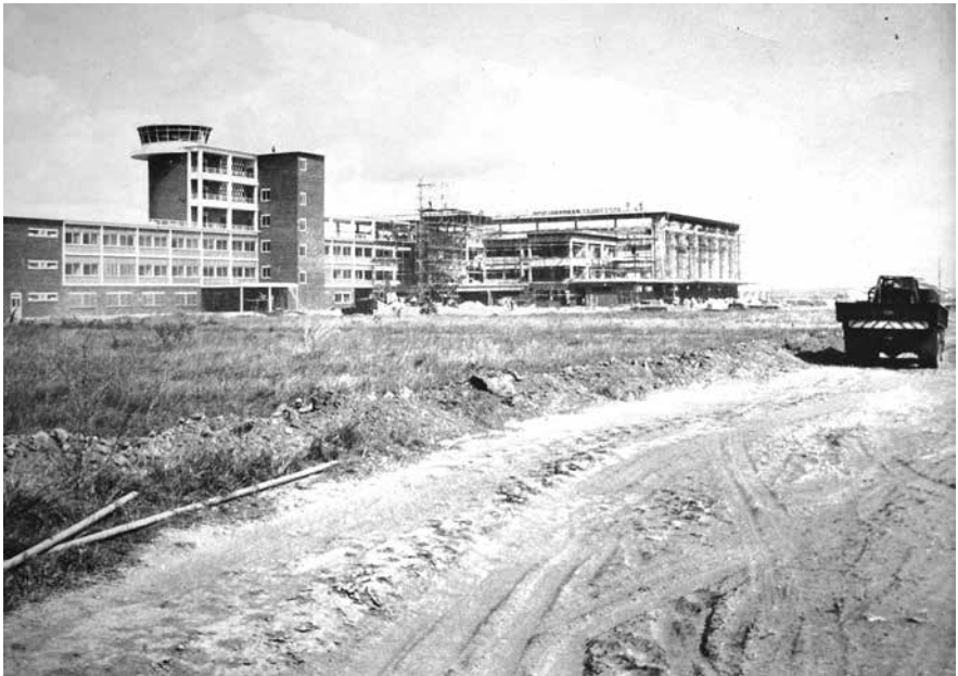
Construction of the new airport approaches completion 1967
