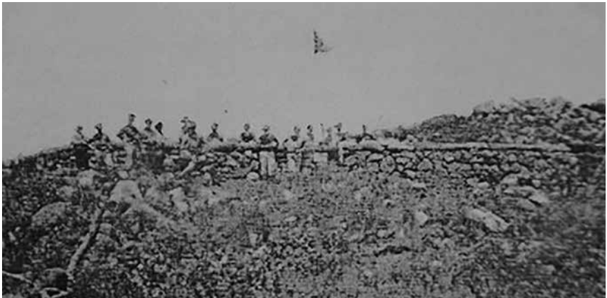
Fort Harding soon after completion – before the corrugated iron store room / command post was erected
