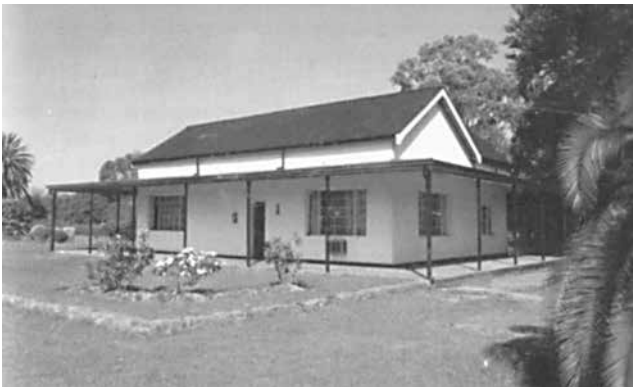
John and Poppy Mack's house (now the Mine Manager's Office).
