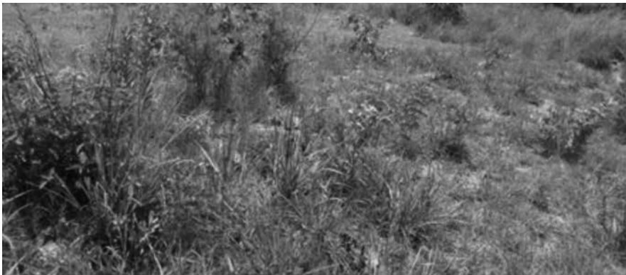
Foundations of one of the Police Camp buildings
