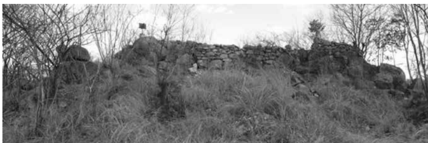
The Fort from below showing the Trig beacon on the left and entrance on the right
