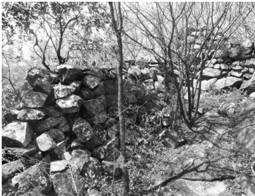
Interior north west wall
