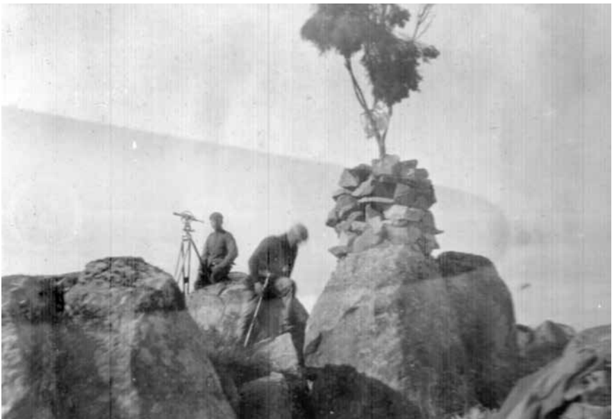
Figure 14: Trigonometrical point at Mount Inyangani, just behind the highest point in Zimbabwe. The pile of rocks is the first boundary marker in the area, now replaced with a more permanent structure made with concrete. (Bulawayo Public Library Collection)
