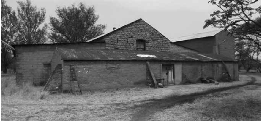
Western view of the Coaching Stables; surrounded on all sides by lean-to additions, note bricked-in rifle-slits
