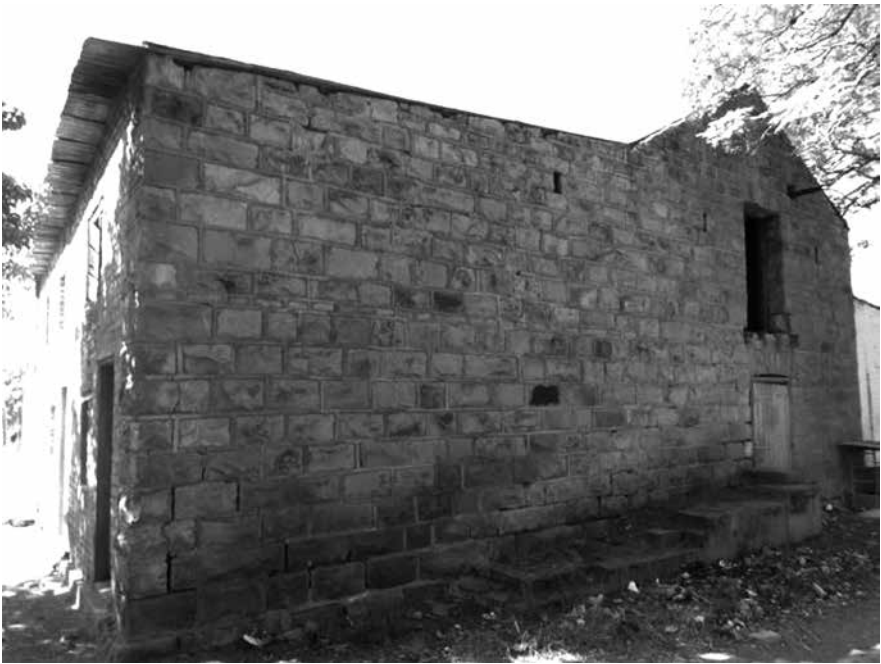
Mill from the west, showing entrance into the loft; note the rifle-slits. The coach bays, now bricked in, are on the left of the photo.
