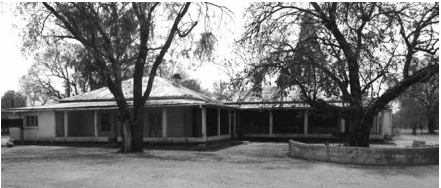
Meikles Hotel from the west showing the covered verandah
