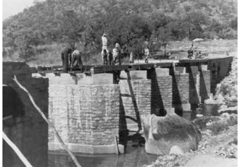
Stephen Peet's first location: Mwaradzi Bridge. This was the title of the second production listed in the 1950 CAFU catalogue. The year was 1948 and the site was the Mwaradzi Bridge.
