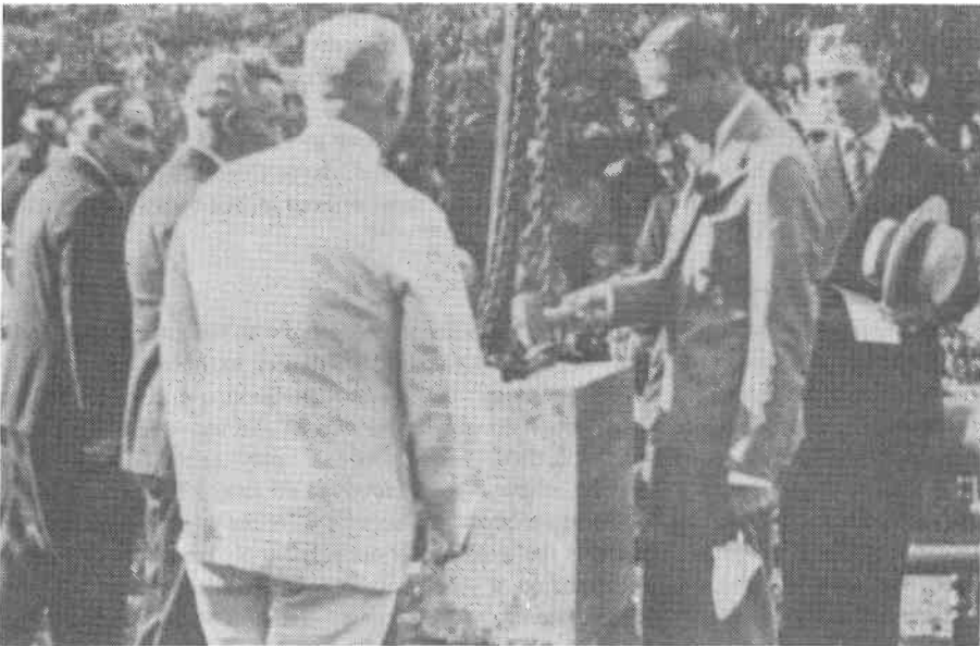
Prince George lays Club foundation stone March 1934
