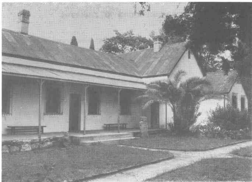
Figure 5. The same view as '4', after renovation. The 1894 structure is on the left; the large gable dates from 1901, and the smaller from 1940 (Photo Ilo)
