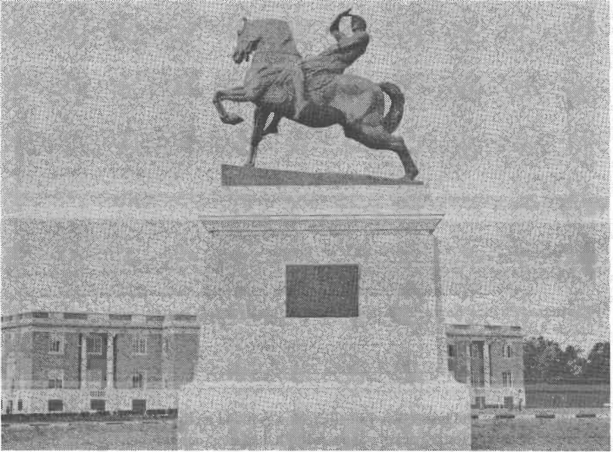
“Physical Energy” in Lusaka showing the High Court in the background, 1960
