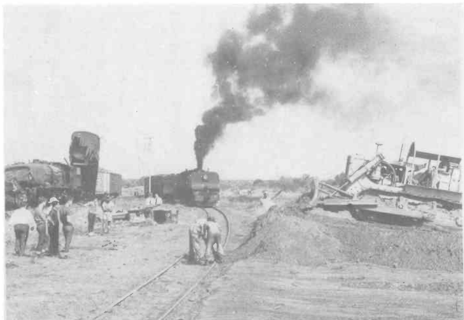
Derailements and washaways were common — here a bull-dozer is seen in the laying of a by-pass track after a serious collision in Botswana, 1960s (Phil Killin)
