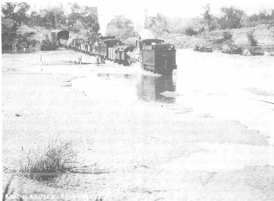
Low level crossing of Shashi river during construction of main line, 1897. Note trucks washed down river in flood. C.G.R. locos on construction train
