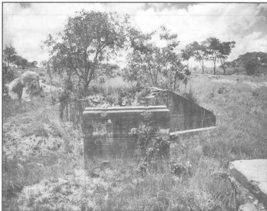
Concrete remains of bridge across Mapfeni river taken November 1997
