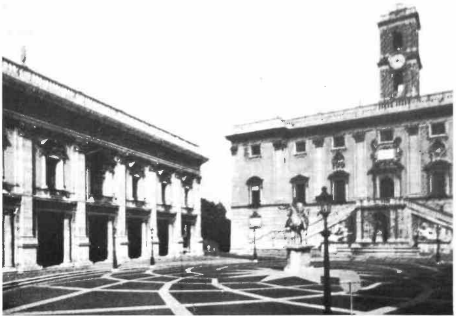
The eastern corner of the Capitol at Rome, to the design of Michelangelo Buonarroti, between 1450 and 1644. The two-storey Capitoline Museum has pilasters with Corinthian capitals and, above the entablature is a pierced balustrade.
