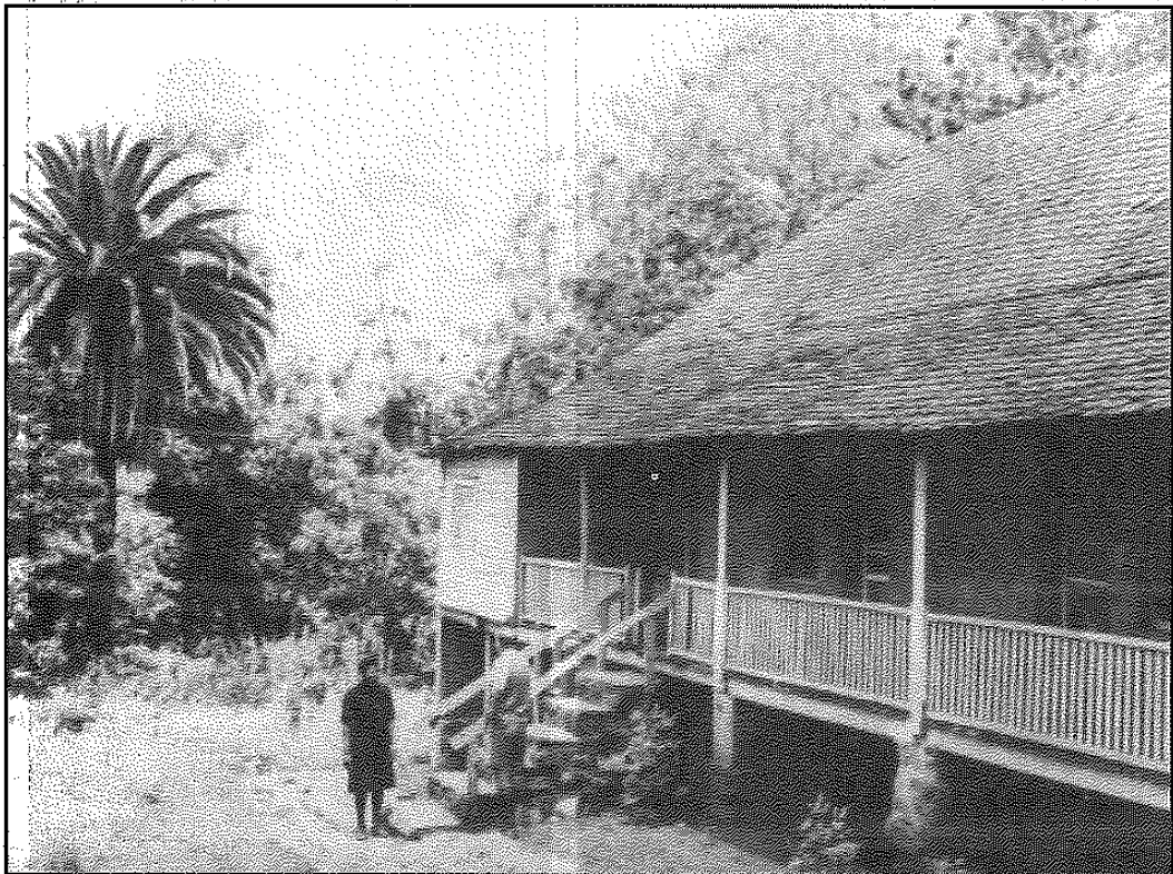
One of the early mission buildings built 1890s on pillars to avoid termite damage.
