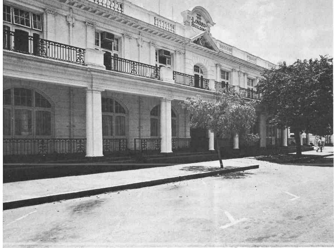
Lonrho Building 1910. Architect J.A. Cope-Christie
