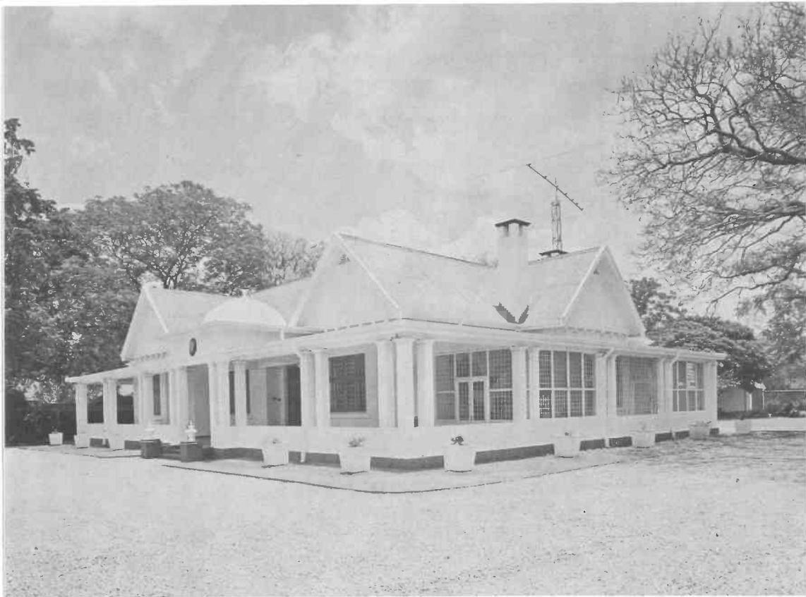
Norwegian Embassy 1923. Architect J.A. Cope-Christie
