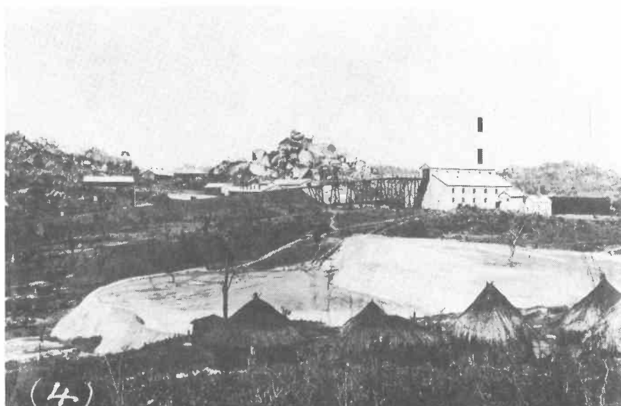
Also taken in 1905 this photograph shows the processing section of the mine which is uphill and some distance away from the Mine Shaft shown in Figure 2. Further Steam engines and the stamps were enclosed in the large prefabricated building right of centre (National Archives of Zimbabwe)
