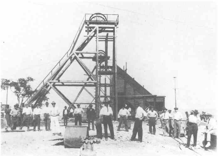
The Head gear of the Edwards Shaft, Ayrshire Mine. Exact date unknown but is likely to be about 1902 soon after its erection
