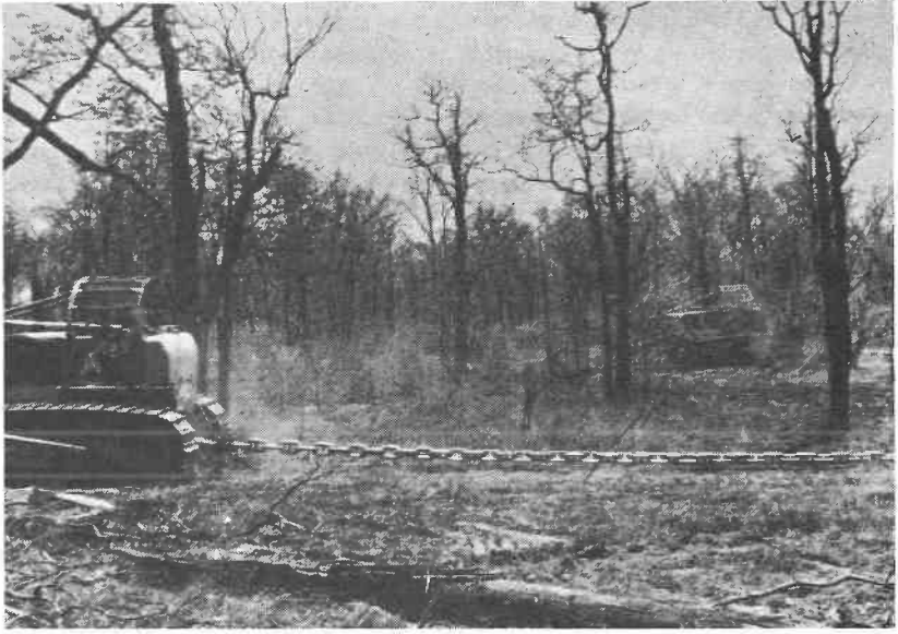
Bush clearing, Kariba basin: 2 tractors with anchor chain between them, October 1958 (National Archives of Zimbabwe)
