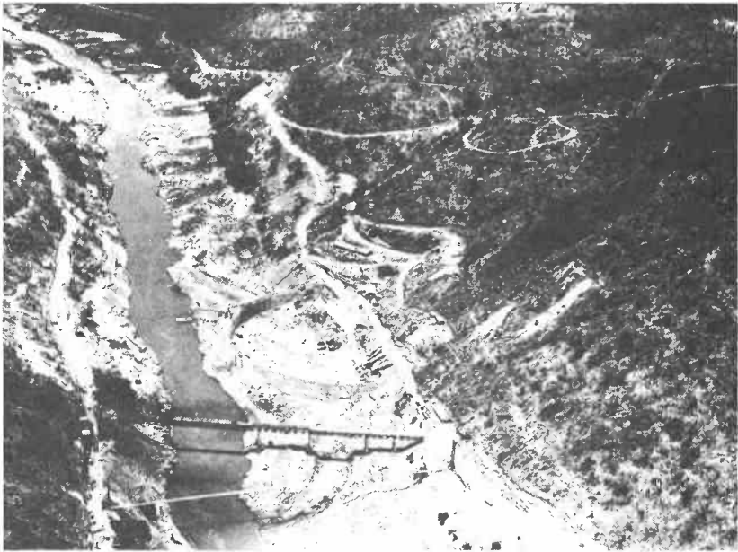
Aerial view showing the first coffer dam, nearing completion, 1956
