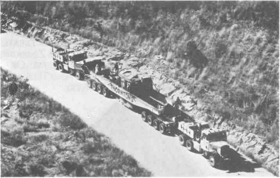
First transformer being moved along Elephants' Path
