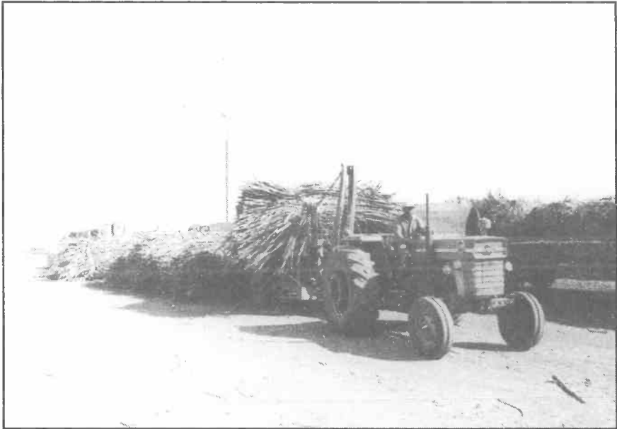
Bundle being offloaded at the train siding
