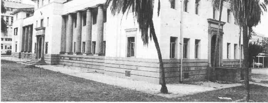
Old Land Bank Building demolished in 1984.
