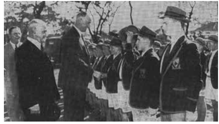
The Governor of Southern Rhodesia, Sir John Kennedy, inspecting the St Joseph's 'guard of honour' on the occasion of his laying the foundation stone of the new House, in July 1951. Mr J. W. Miller, Chairman of the General Committee (far left) and Major A. I. Rice, Warden, are accompanying the Governor. [Photo: The Rhodesia Herald ]
