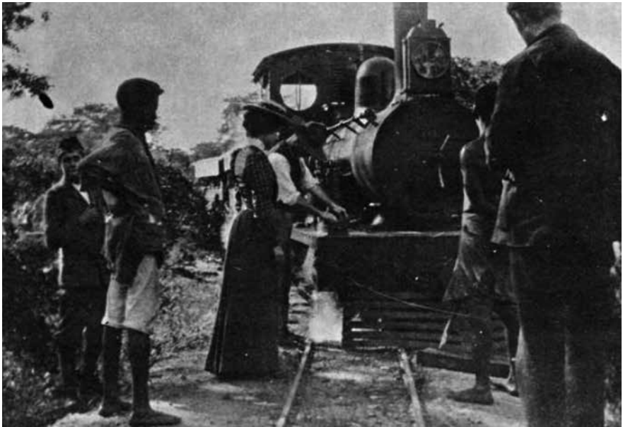
The narrow gauge engine has come off the line—a fairly frequent occurrence.
