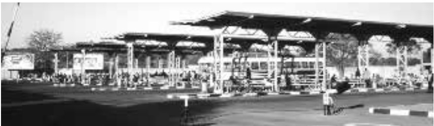
The modern bus station at KweKwe in August 1984, with an AVM vehicle of Hall & Son. The station was located at Amaveni Township, rather than the main town centre
