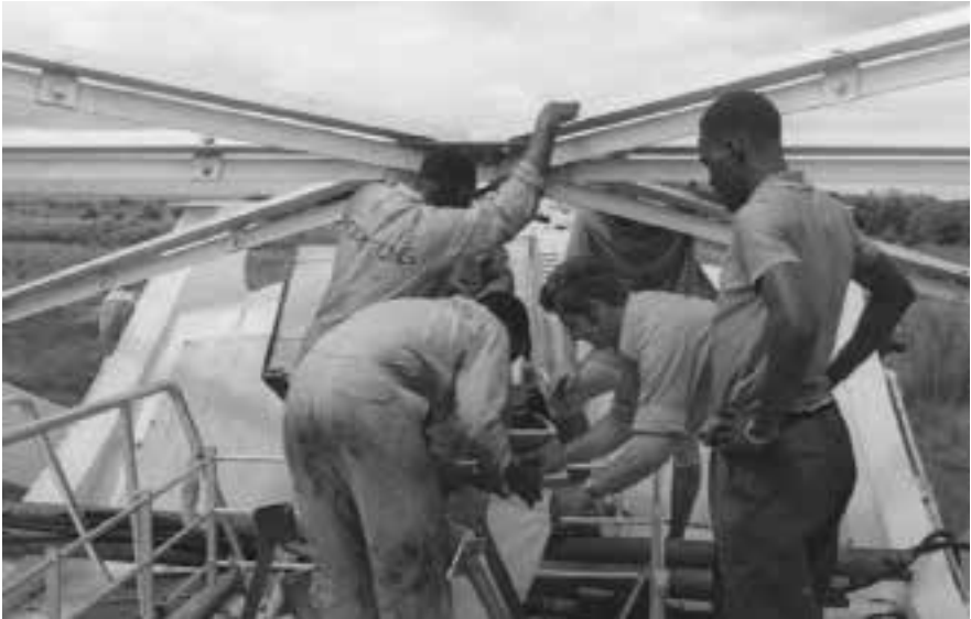
Trying to loosen the top girders of the bridge. Bev Portman (leaning forward) and his team, working from the deck of the hydrofoil, parked, as far as it could go, under the bridge.
