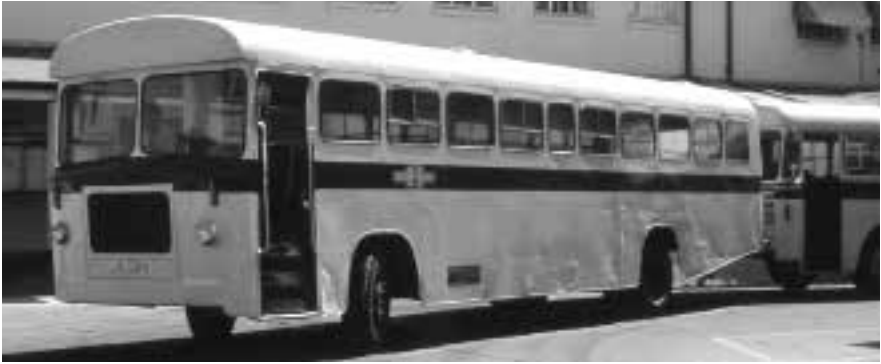
An older Leyland single-decker of the Zimbabwe Omnibus Company used on Bulawayo urban services in 1984. Note the front entrance and high floor level.
