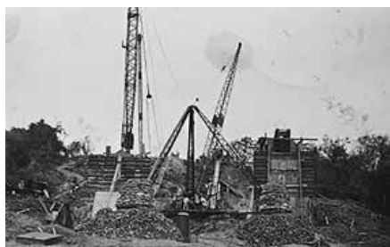
Fig. 2. Laying of the east bank foundations.
