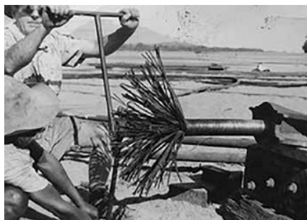
Fig. 7. Refabricating the Sydney Harbour Bridge cables to support the roadway.
