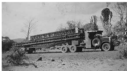
Fig. 3. RMS lorry transporting sections of the steel framework of the bridge from Umtali to the construction site.
