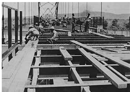
Fig. 6. Constructing the suspended roadway.
