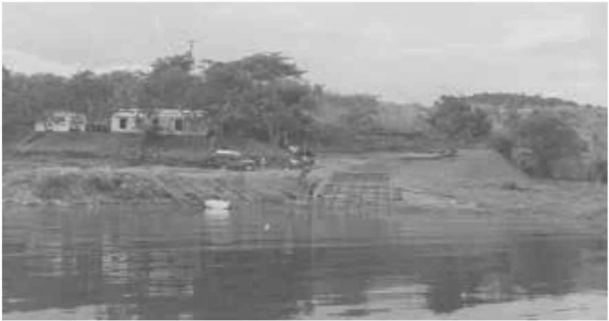
Taken early in 1972, showing the slipway under construction, the prefabricated office cum stores building and the staff caravan.
