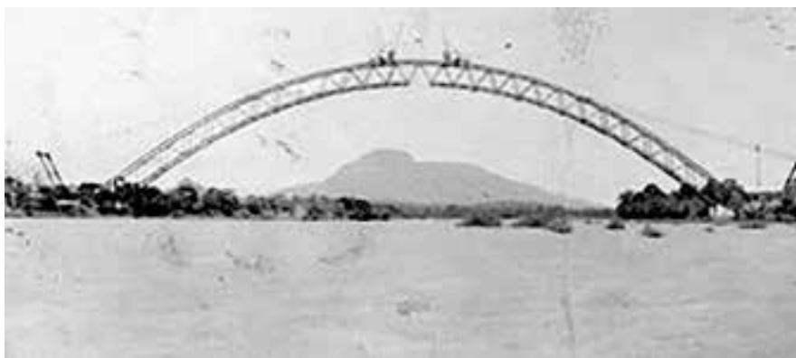
Fig. 5. The arch completed, 17 June 1935.
