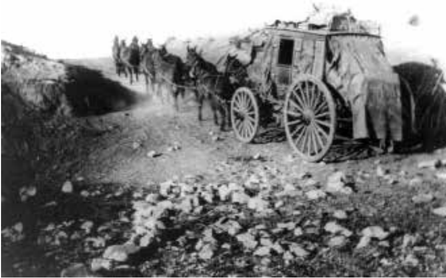
Typical Road Conditions (note the rocks)
