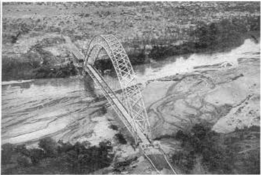
THE BIRCHENOUGH BRIDGE across the Sabi River, Southern Rhodesia, which will be opened to-morrow. The third largest single-span bridge in the world, its arch rises 280 feet above the river, and it is 1,080 feet long. It was made by British contractors.
