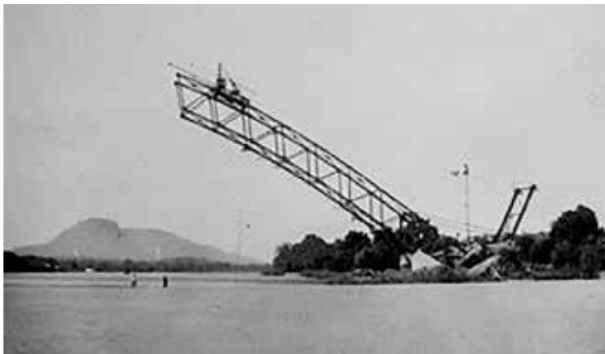
Fig. 4. The west bank portion of the bridge being erected outward supported by “Sydney Harbour” cables.
